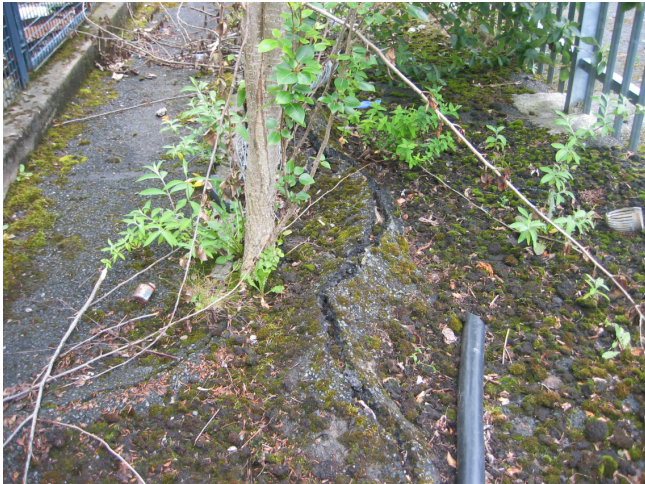
Photo 7: Signs of root damage to paved surface
